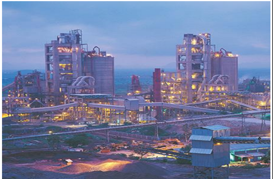
Figure 39: JKLC's integrated plant at Jaykaypuram, Sirohi (Rajasthan)
